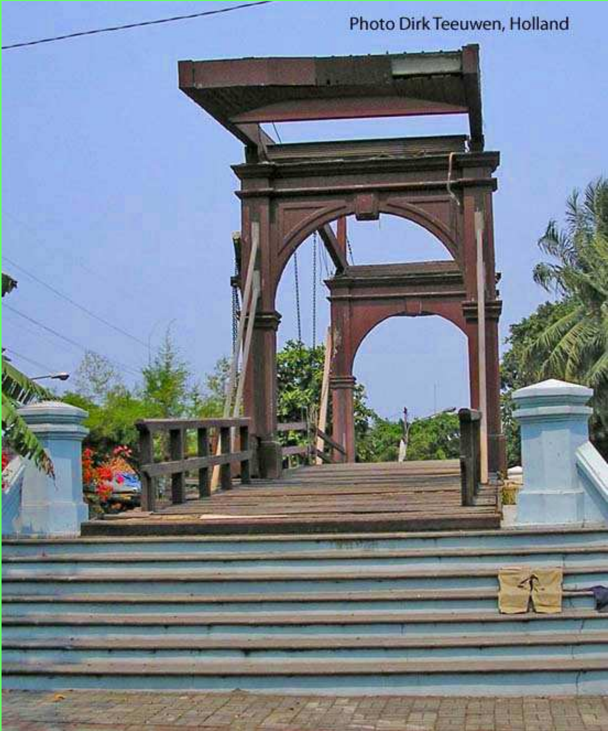
1 Jembata Kota Intan, Old Diamant Bridge in 2006
